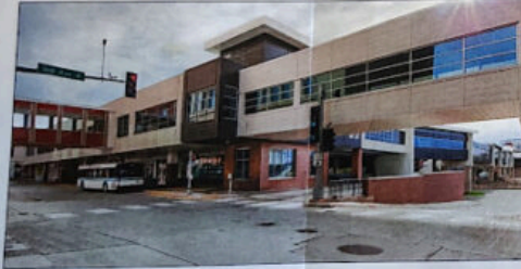
Duluth Transportation Center | Completed 2016
